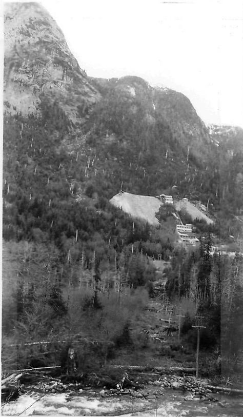
Plate 1: Surf Inlet Consolidated Gold Mine Limited, 1935; production from 1902 to 1943, 1 million tons, 389,000 ounces. A typical north coast mining operation. Quartz veins within sheared zones in gneissic quartz diorite.
