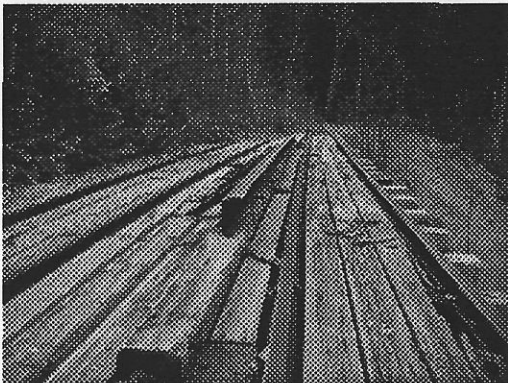
Rail Dump At 1025 Portal
