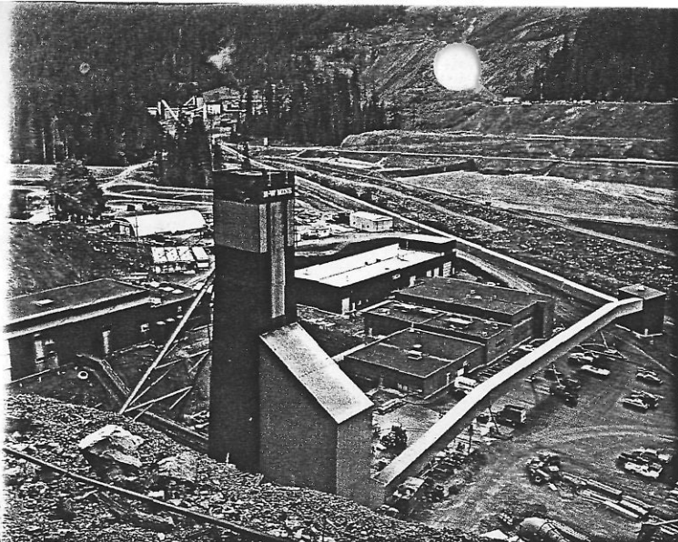
Westmin's H-W headframe, shops and office buildings with conveyor taking ore to the mill in the distance.
