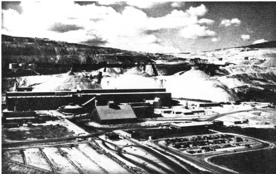
Aerial view of Highland Valley Copper mill, Logan Lake, B.C. A-frame building in foreground is copper concentrate storage and loadout point.
