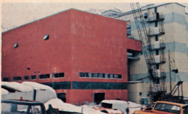
Cassiar's new mill air building provides 480,000 cfm of process and ventilating air.
