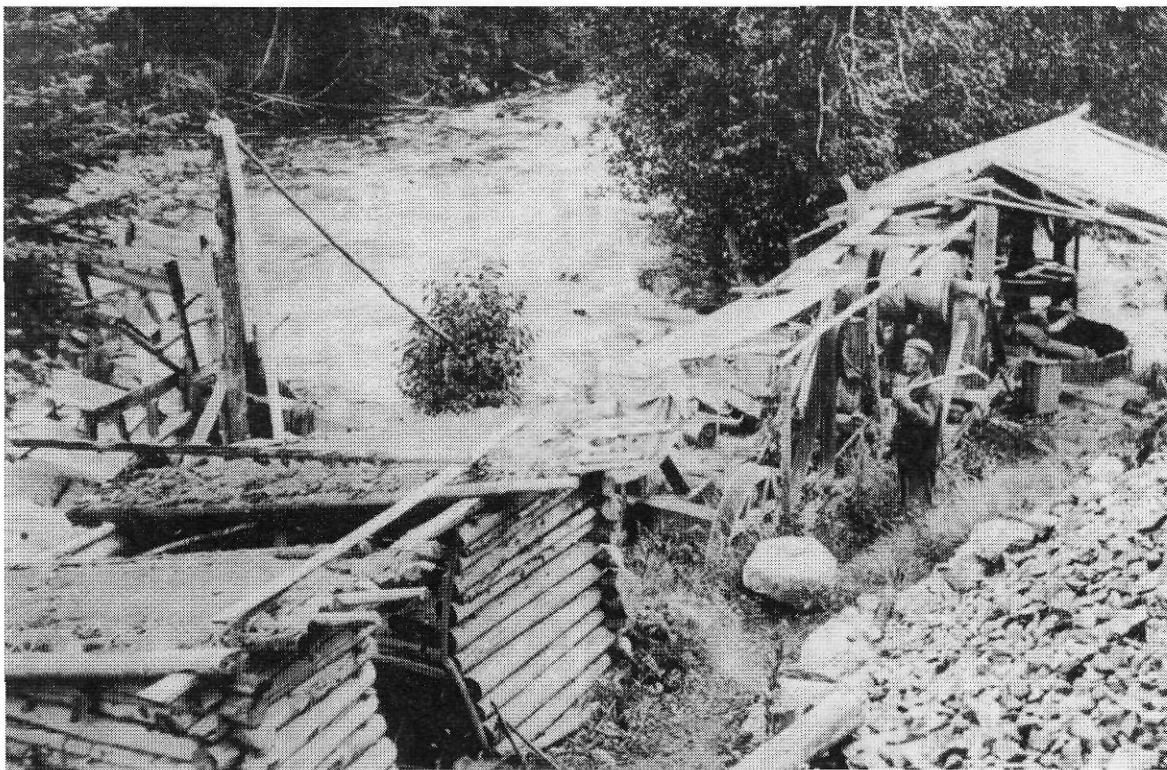
Fred Kinder's "one-man mine," on Cadwallader Creek, which eventually became part of the Bralorne holdings. The water-powered arrastra shown here was the first mill in the district. Primitive though it was, it was a considerable improvement over Kinder's mail-order stamp mill.
