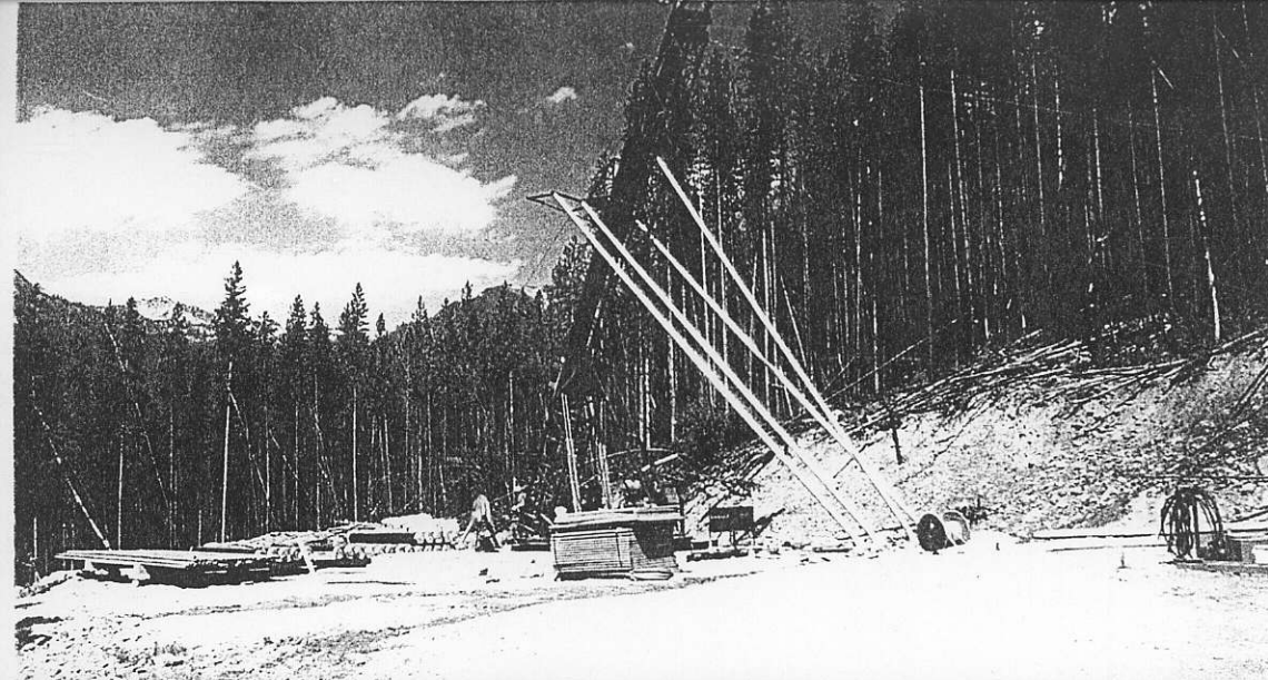
10. Tower raised support leg and guide cables in place.
