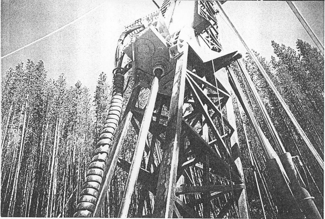
21. Lower section of tower with drill head in raised position.
