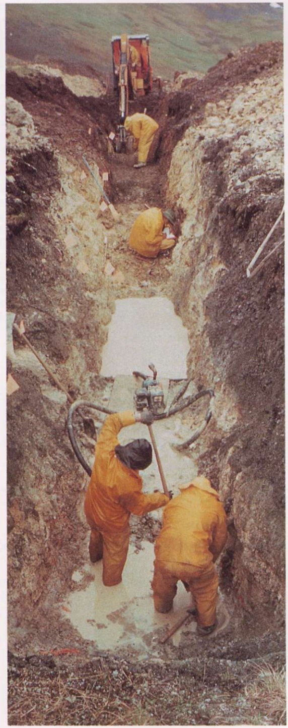
Typical Backhoe Trenching and Surface Sampling
