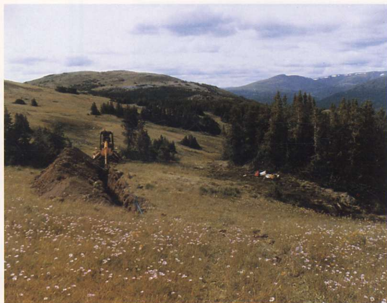
Backhoe trenching, AI Property, Albert's Hump in centre background.
