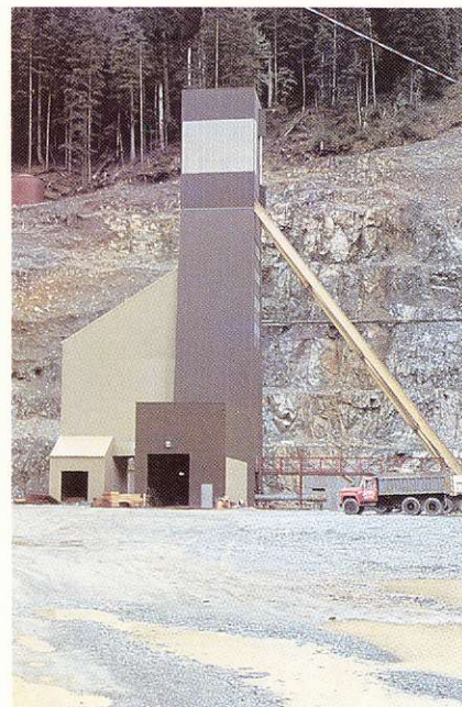
The new H-W headframe over the shaft which is down to 1,370 feet. Lateral work, more diamond drilling and bulk sampling will precede sinking to 2,500 ft. target depth.
