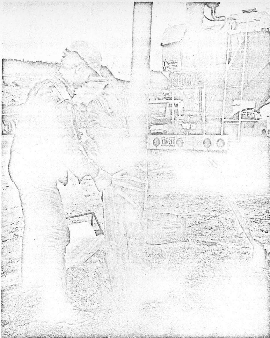
Mixture of ammonium-nitrate prills and fuel oil is pumped into blast holes
