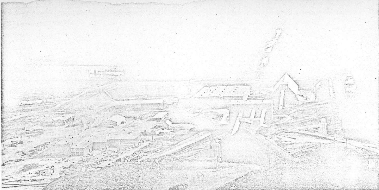
The Gibraltar concentrator complex as it appeared in March 1972. Primary crusher building and coarse-ore stockpile are visible in centre foreground. Secondary-crusher building is directly behind the coarse-ore stockpile. Fine-ore storage is covered by A-frame structure at right with main concentrator building to its left. Shop warehouse and garage are housed in the big building in left foreground.
