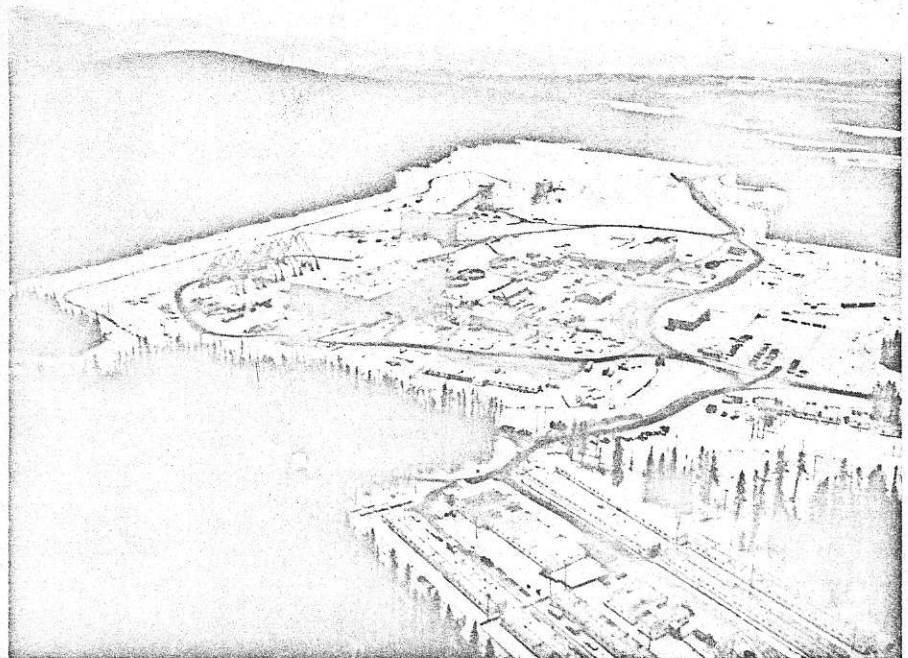
View of Gibraltar plant site, looking S.S.E. Concentrator is visible in centre with A-frame fine-ore storage bin taking shape to left. Gibraltar East pit is visible as cleared area at extreme right, beyond trees.
