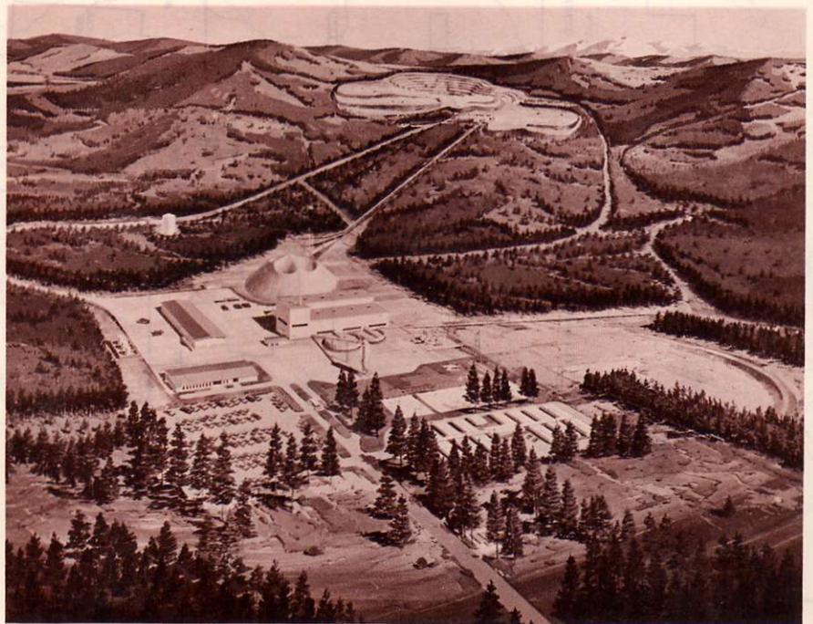
Artist's conception of Lornex Mining Corporation's planned open-pit copper mine. The development is estimated to cost \$120 million and, the company states, it will be the largest single mining operation in Canada. The sketch shows the open pit (background), coarse-ore stockpile, mill building, repair shop, administration building, and mine camp.
