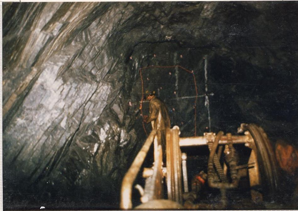
PLATE IV: Mucking machine in 10820E crosscut dumping waste material into ore car for removal from the underground workings.
