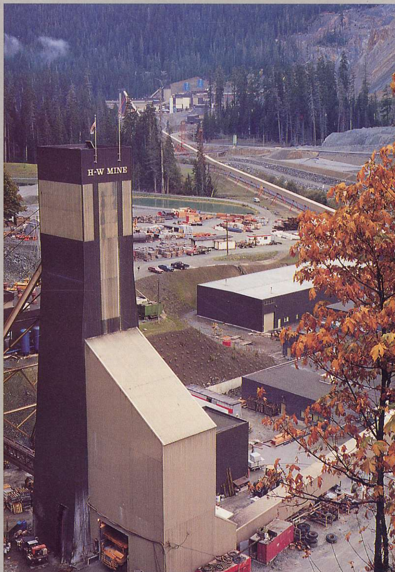
Overlooking the Myra Falls complex with H-W headframe in foregoing and mile-long conveyor taking ore to the mill.
