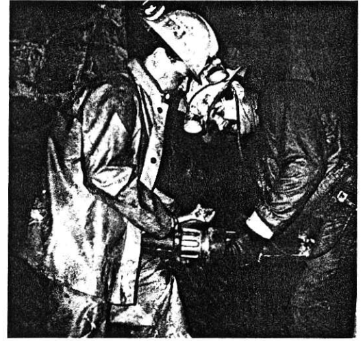
Miners working underground on the Lara project's 600 level.
