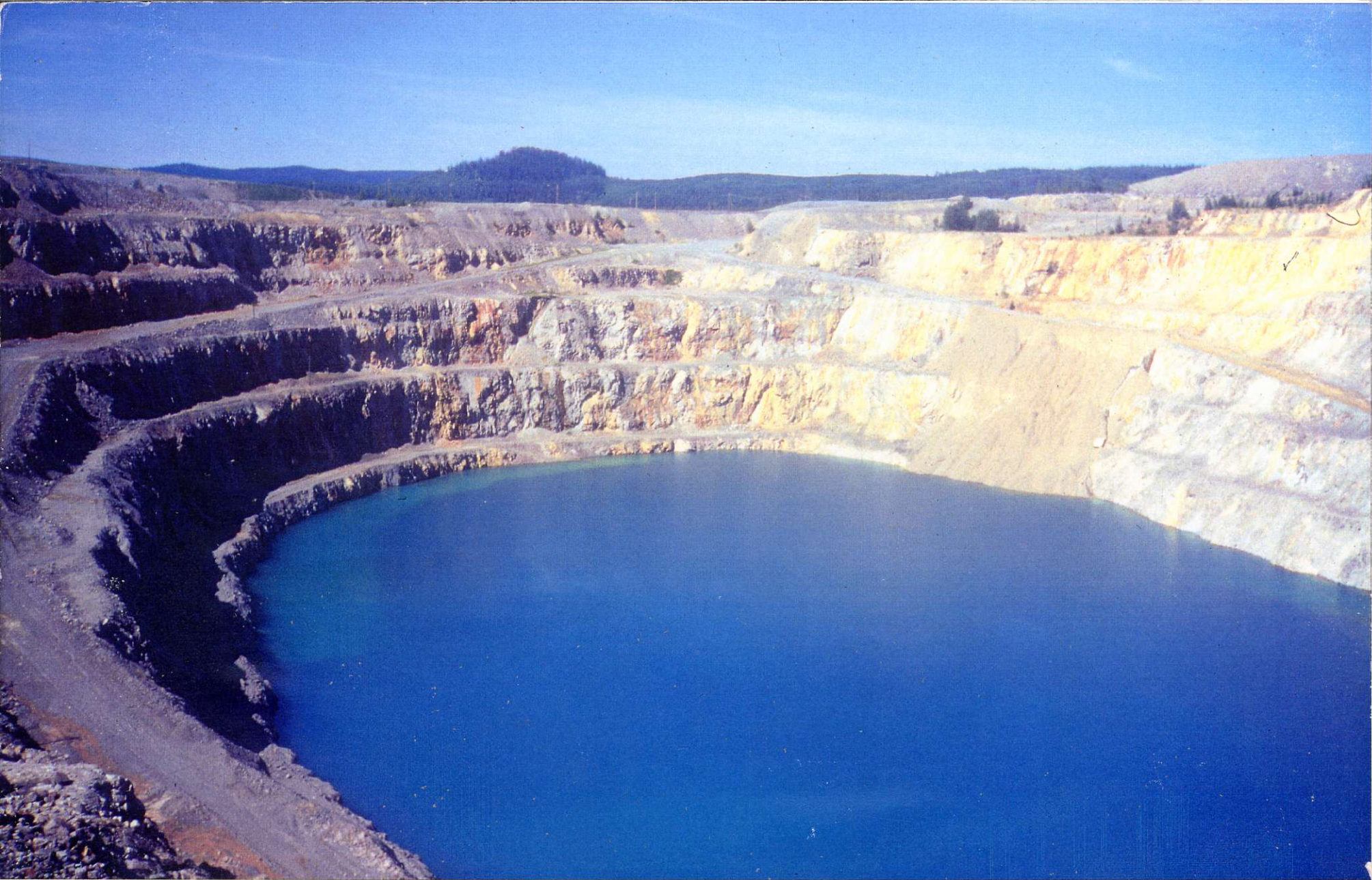
View looking northwest across the Granisle open pit. The Granisle mine produced 214 300 tonnes copper, 6 833 kg of gold and 69 753 kg silver from 52.7 million tonnes of ore between 1966 and 1982. Copper occurs within and peripheral to biotite-feldspar and quartz-biotite-feldspar porphyry intrusions of Eocene age (EBp).
