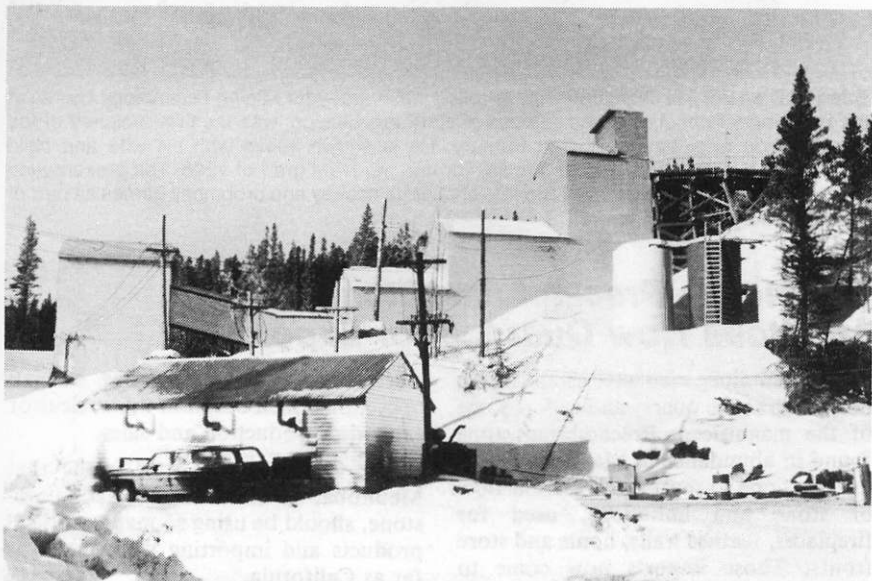
The 150-ton-capacity mill at the Erickson Creek gold mine.
