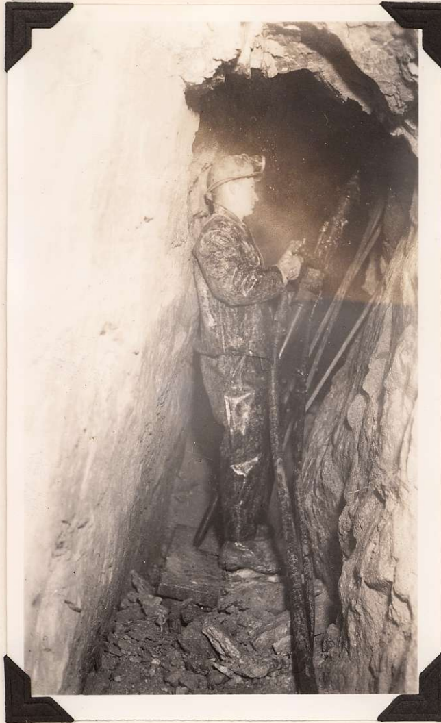
Striations on Hangingwall - Showing Movement - But No Displacement of Vein 4 Level - 58 Stope
