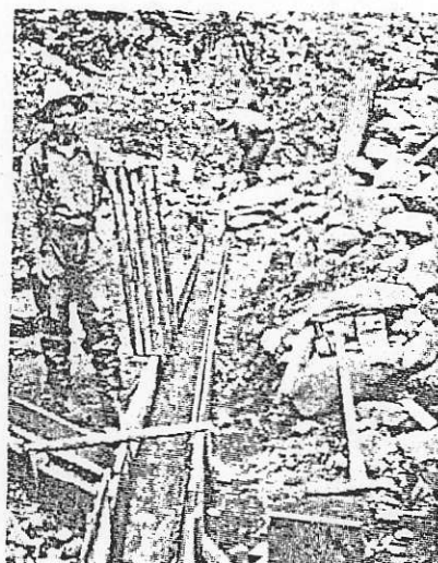
Figure 21. Miner Holding a Frame of Riffles. The removeable tray allows for easier cleanup. [from Basque's " History of the Canadian West ," November 1983, p. 99]
