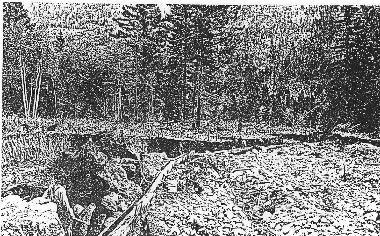
Figure 19. A Sluice Used at North Bend, British Columbia. Reports do not indicate that such a long sluice was ever used at Goldstream. [from the British Columbia Provincial Archives, #77719]
