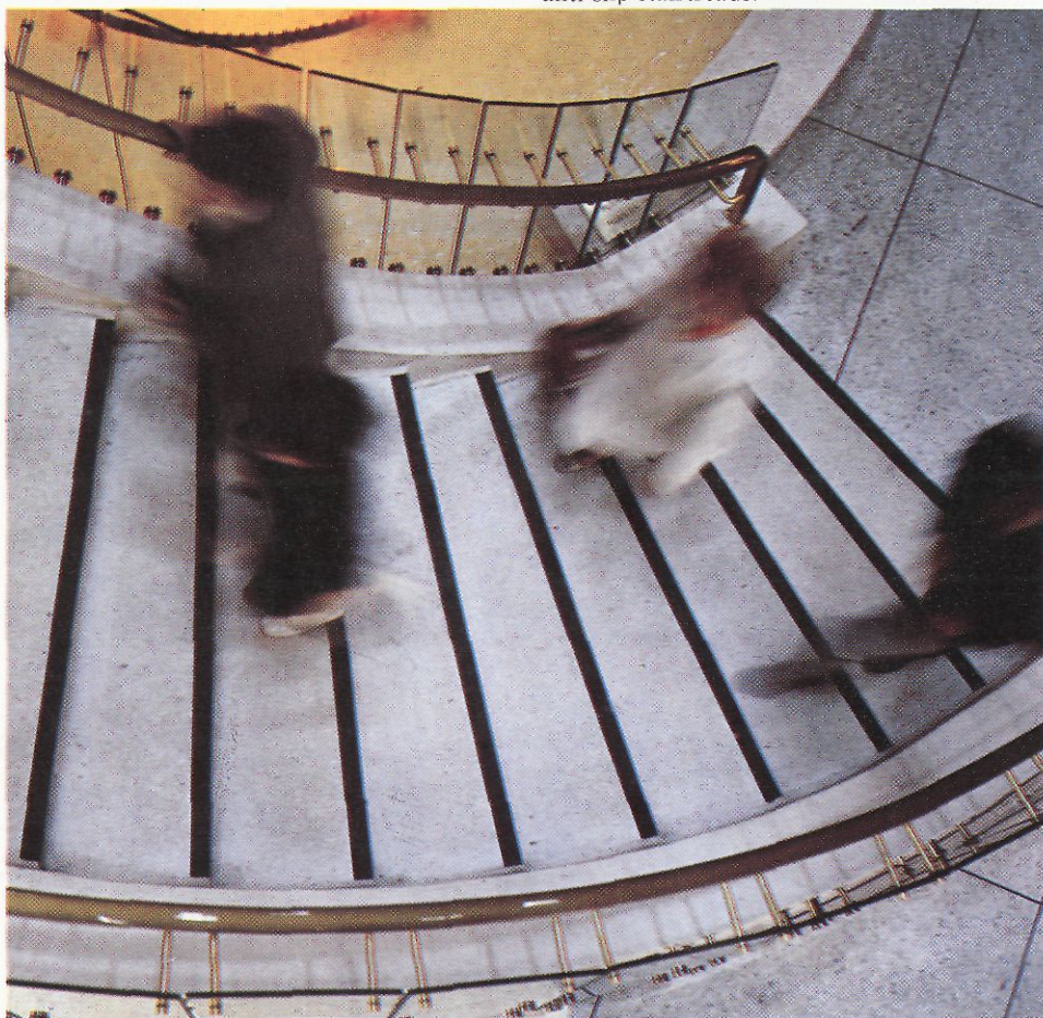
29 Asbestos-based friction material is incorporated into anti-slip stairtreads.
