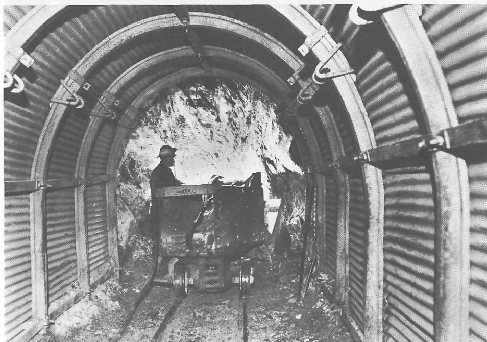
17 An underground gallery at Bell Asbestos Mines Ltd., Thetford Mines, Quebec, showing the use of yieldable arches.
