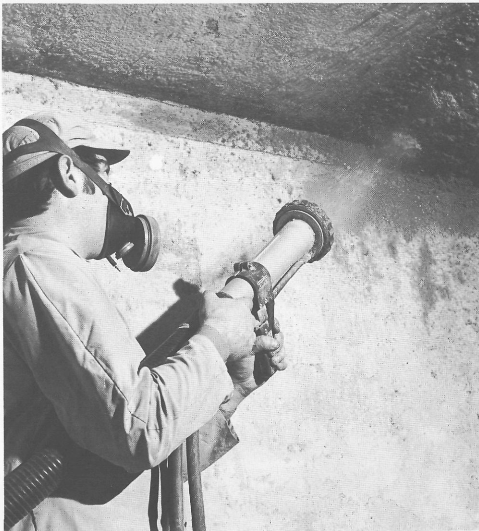
37 The application of sprayed asbestos. Photo: County Studios Ltd., Leigh, Lancs. (GB).
