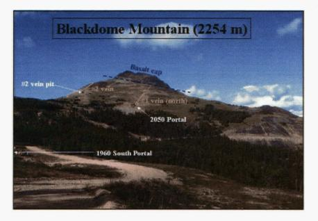
Figure 5 - View of the northern portions of the #1 and #2 veins of the Blackdome vein system beneath the basalt cap, on the south flank of Blackdome Mountain (view looking north).
