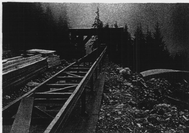
Beginning of construction phase of conveyor system.
