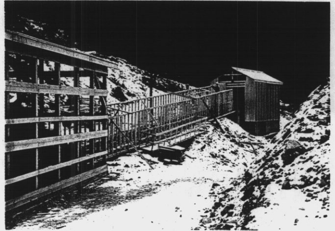
Construction of enclosure of conveyance system.
