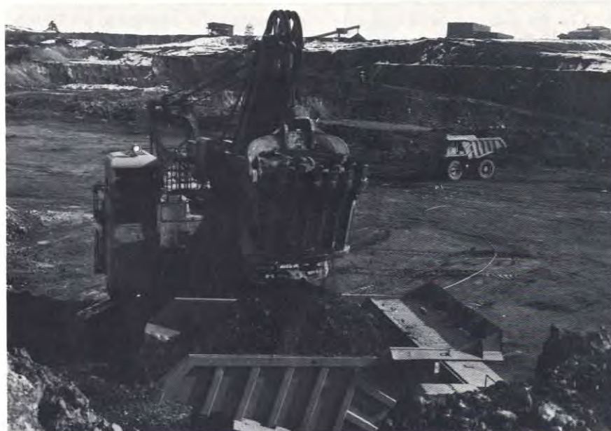
SHOVEL LOADING haul truck with native copper-chalcocite ore. Background, left to right: primary crusher, coarse ore stockpile, concentrator, and maintenance building.
