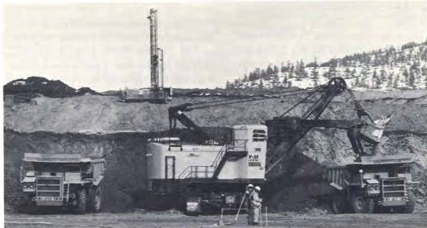
AFTON MINE P&H 1900AL shovel loads one of two Unit Rig 100-ton Lectra-Haul trucks, while Bucyrus Erie 40R drills 9-inch holes in 24 by 24 foot pattern in the background.
