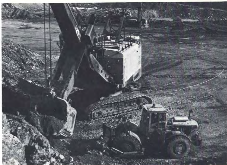
CLEAN-UP around the shovels is accomplished using Caterpillar 824 wheel-type dozer. The final 900-foot deep Dominion pit will cover an area 2,700 by 2,800 feet.
