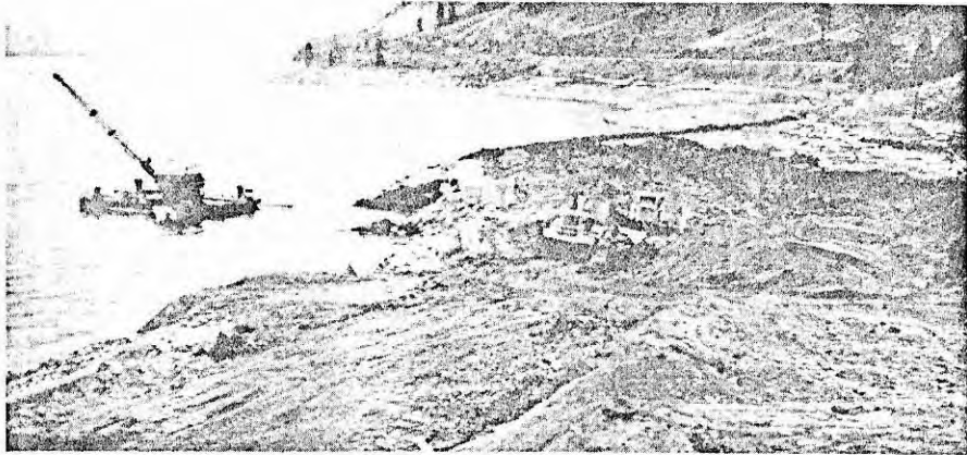
Excavation for pumphouse foundations at Kamloops Lake
