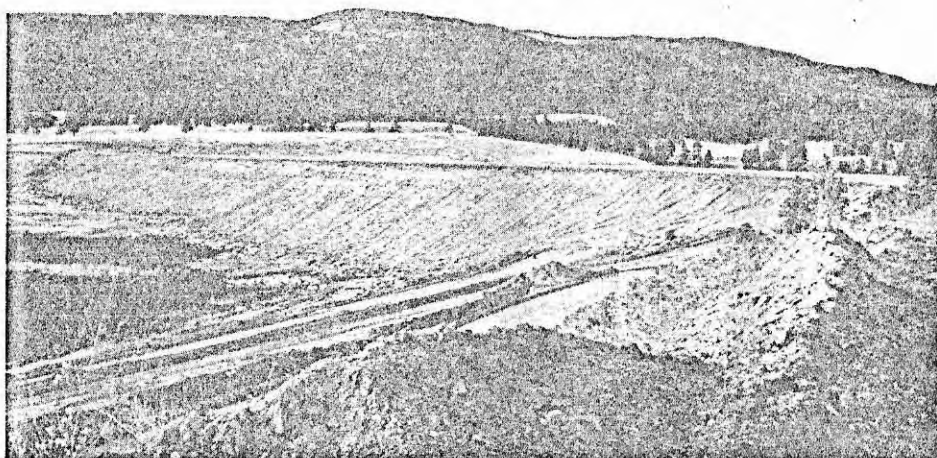
West starter dam prior to tailings discharge
