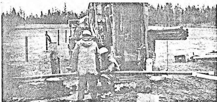
Installation of groundwater monitoring wells
