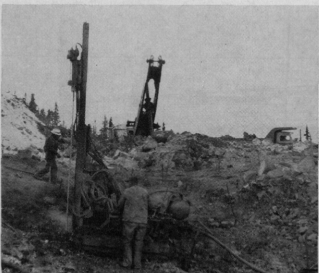
Air Trac machines drilling blast holes to take the top off copper orebody.
