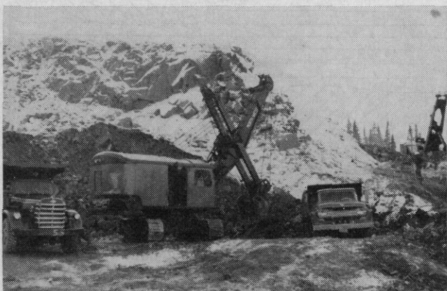
Contractor's equipment includes 1½ cu. yd. shovel and fleet of trucks.
