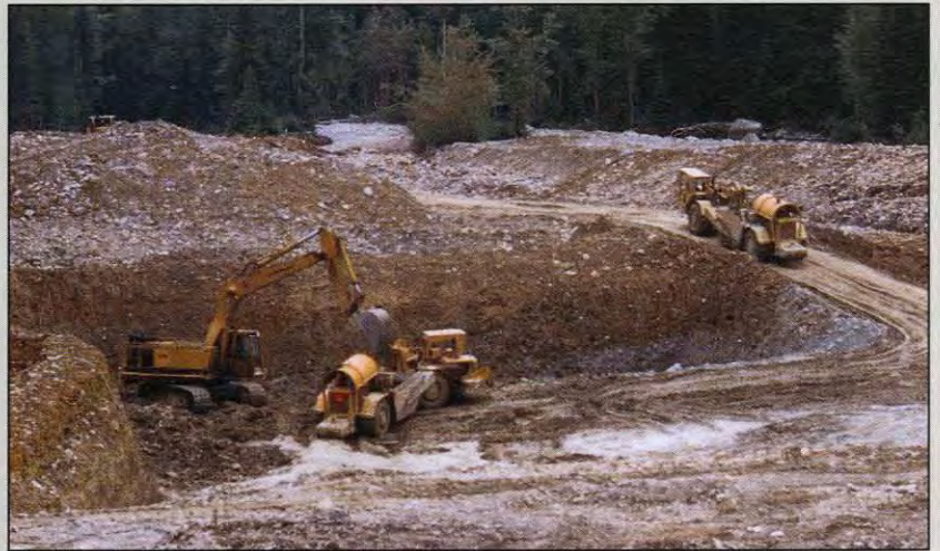
At Moyie River, a 3.75 cubic yard excavator loads scrapers which haul the ore to the gold recovery plant.
