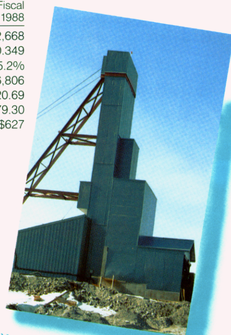
New headframe at the Ptarmigan Mine provides access to potential ore reserves to a depth of 2,200 feet below surface.
