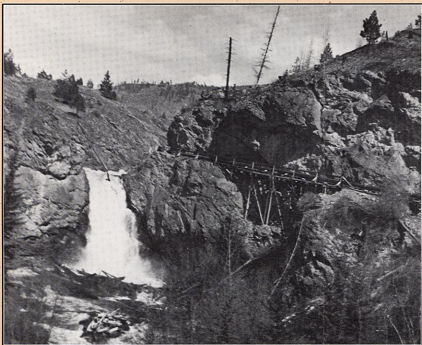
(Left) Looking down on Boundary Falls soon after the pipeline and power plant were constructed. Remains of the cribbing still hang on the canyon wall.
