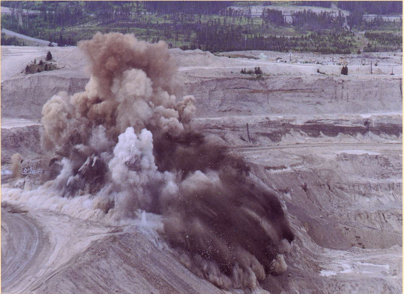
(Top left) The 172 tonne trucks continually feed Valley pit ore into the in-pit crushers. (Top right) Ore from the Lornex pit is crushed in a fixed crusher, which is part of the overall conveyor system. (Above) Production blast in the Valley pit.
