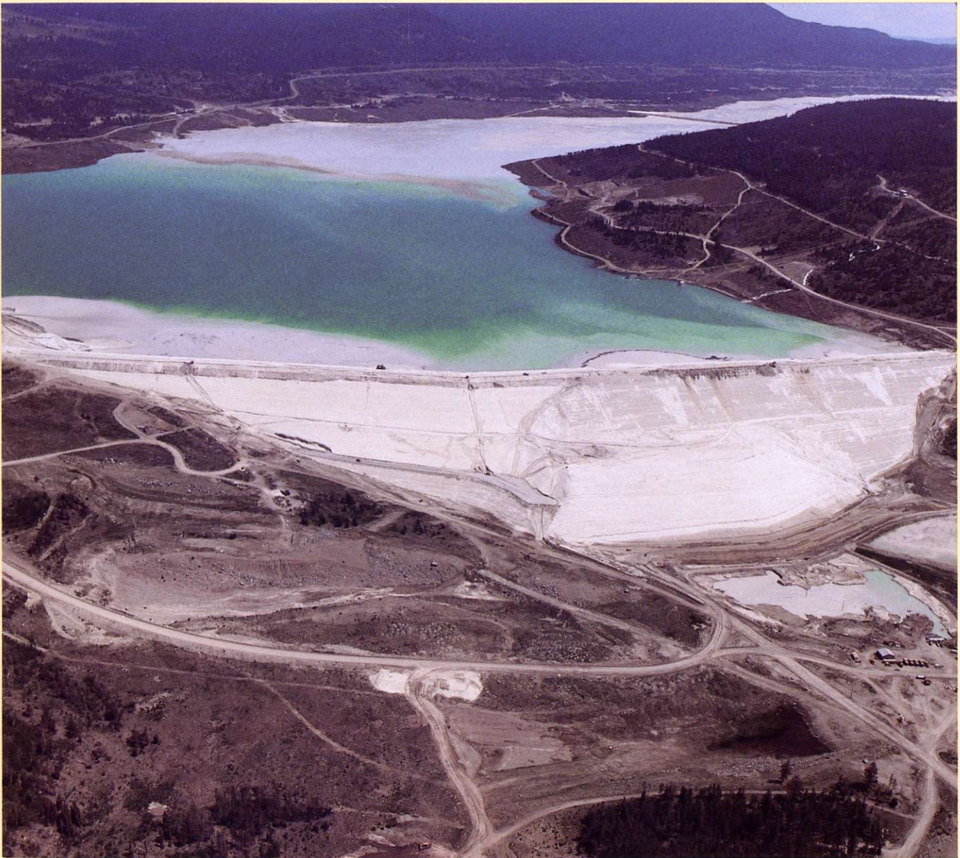
View of the large L-L dam.
