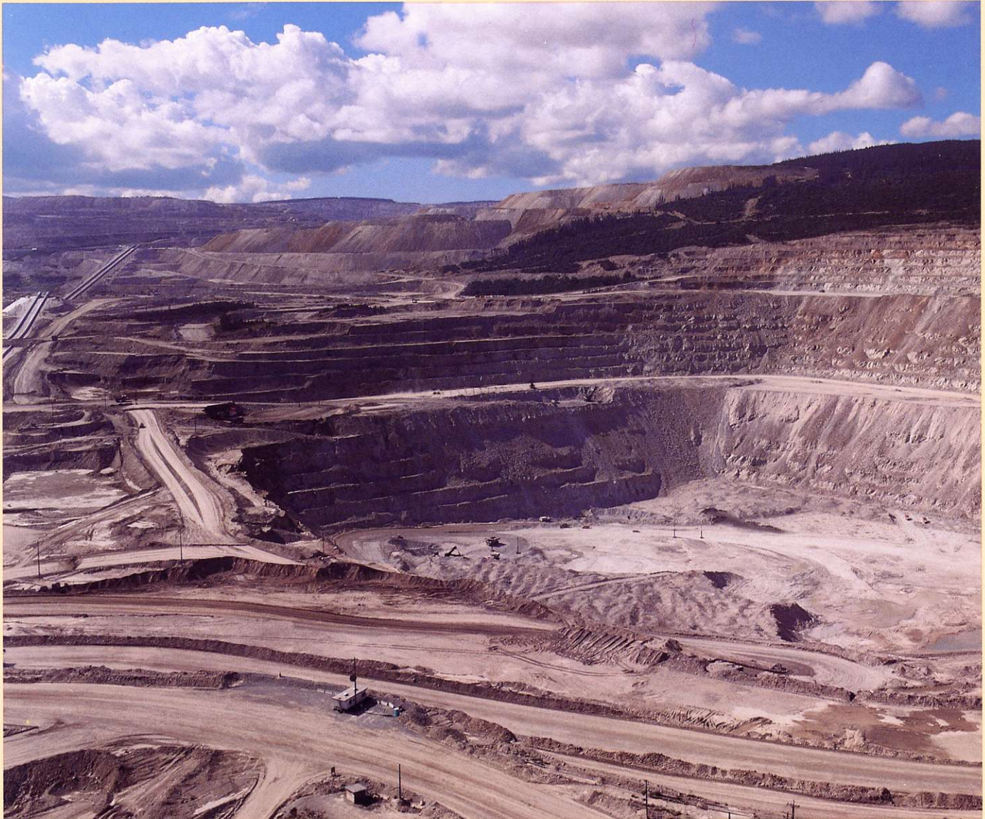
The Valley pit, with the computer controlled dispatch centre at lower left and the conveyor system at upper left.
