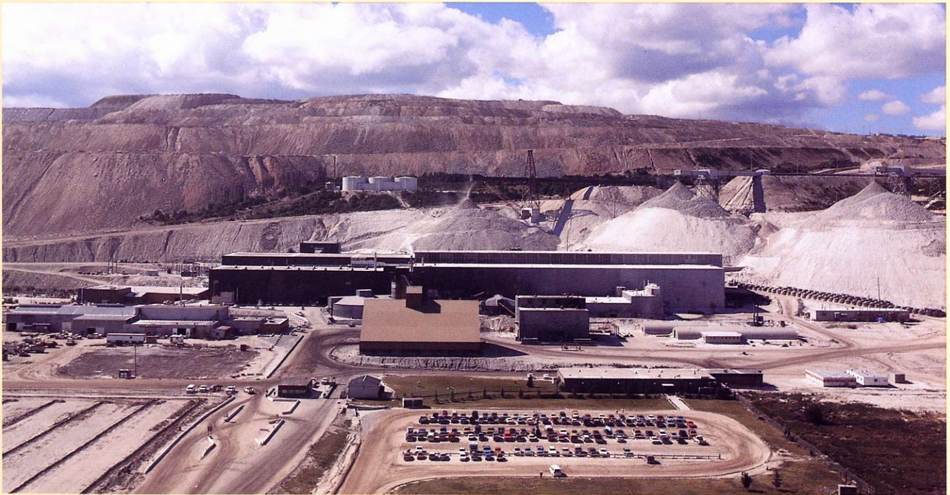
(Top left) The Highland mill with its five grinding lines. (Top right) Repairing the lining of one of the ball mills. (Above) The Highland mill with the concentrate storage shed and molybdenum building along the side (centre right) and the mine administration building (lower right).
