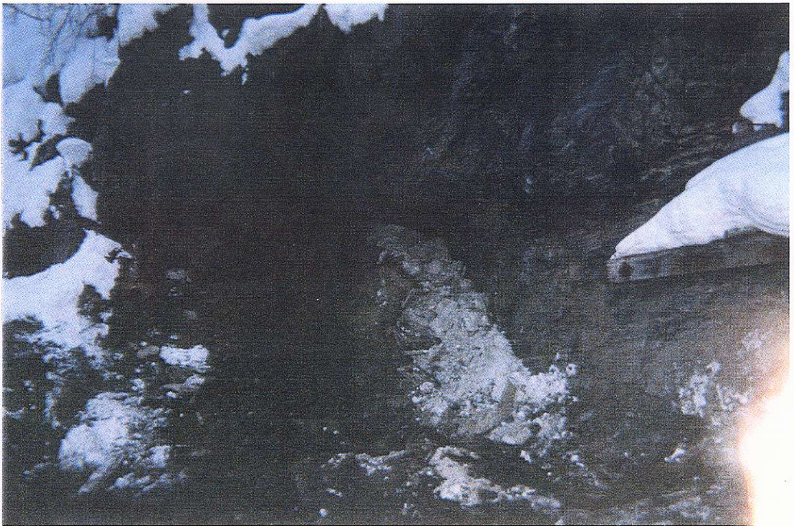
Photo 4: The portal completely sealed with soil and boulders
