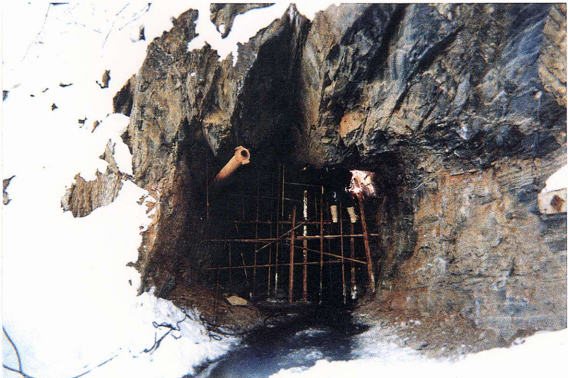
Photo 2: Resealing the portal with iron bars
