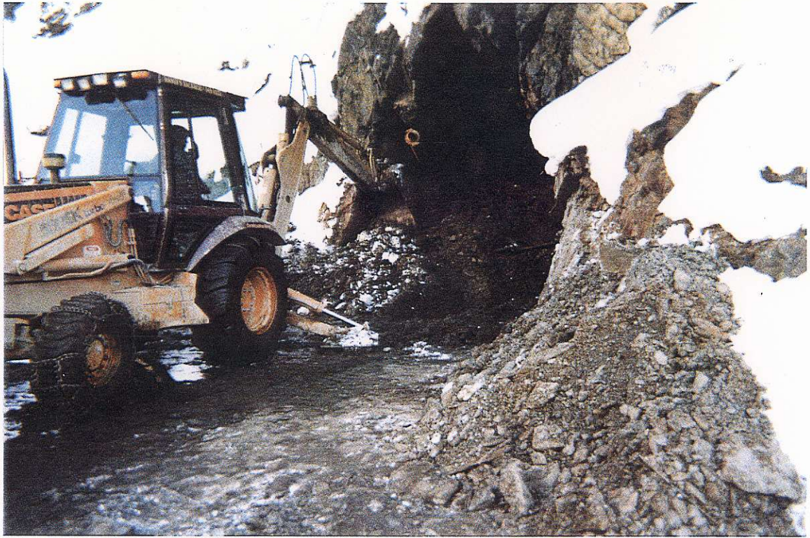
Photo 3: Sealing the portal with soil and boulders
