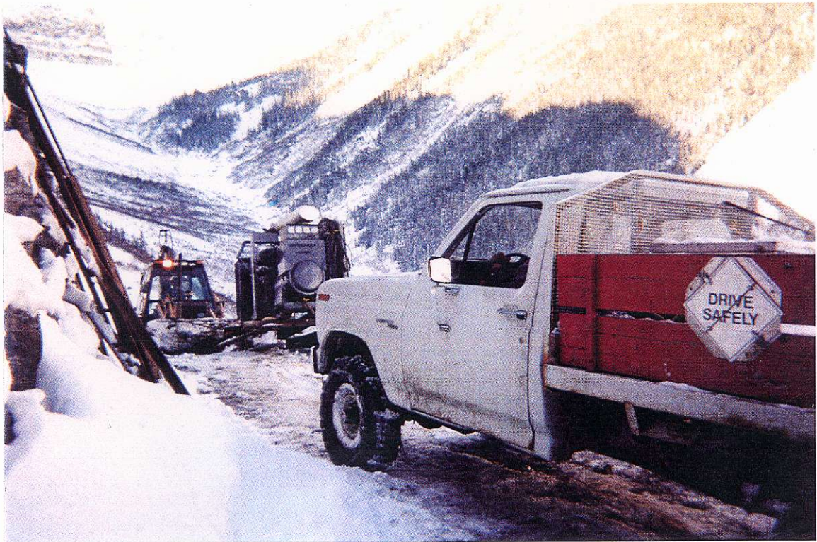
Photo 1: Removal of machinery and equipment from site
