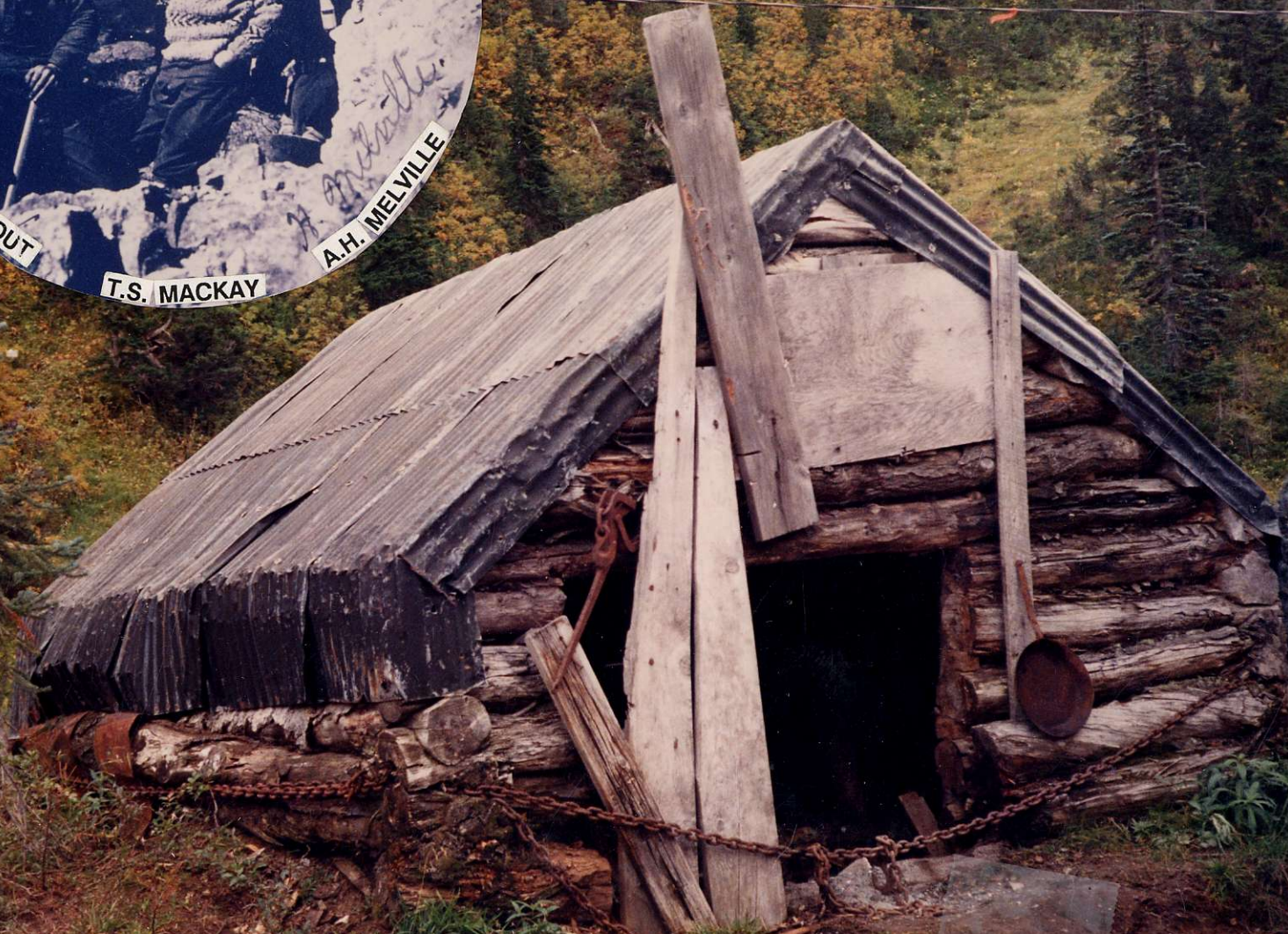
TOM MACKAY'S CABIN, EST.1936 (September, 1989)
