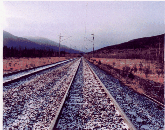
Existing double track at proposed loadout
