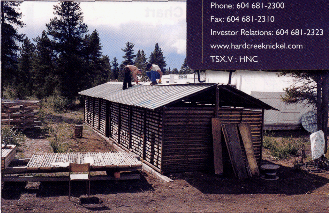
Building Core Shack
