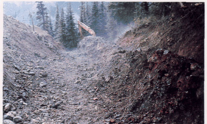
Backhoe trenching on the eastern extension of the Treasure Mountain fault
