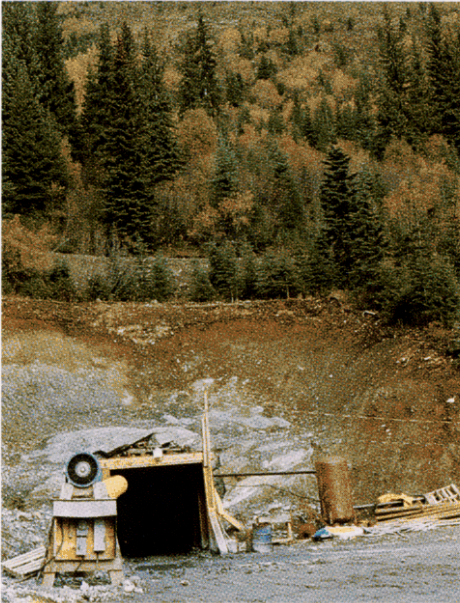
No. 3 level portal with mine road to No. 1 portal shown near top of hill
