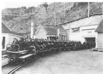
Sullivan mine portal
