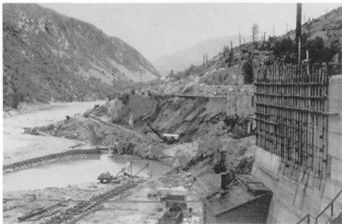
Brilliant Dam construction
