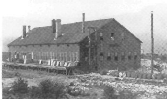
early lead refinery exterior
