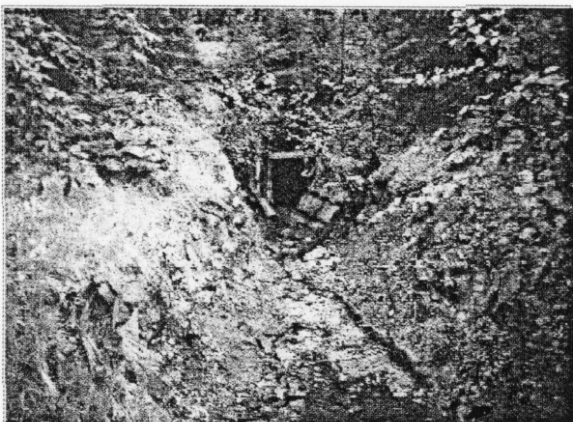
Windpass portal and drainage
