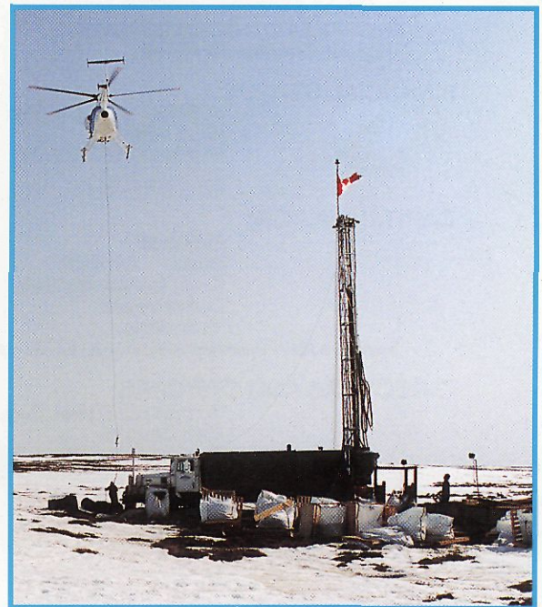
Bulk sample drilling on DO18 pipe.
