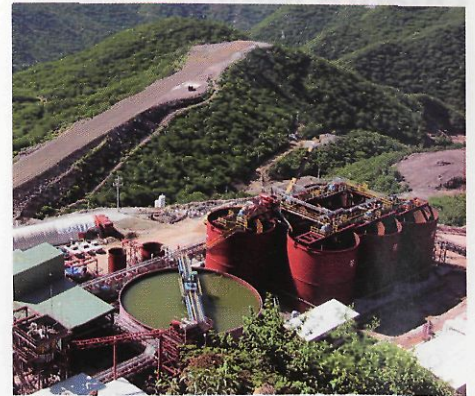
The El Sauzal Mine in Chihuahua state, Mexico. Photo courtesy Glamis Gold Ltd.
