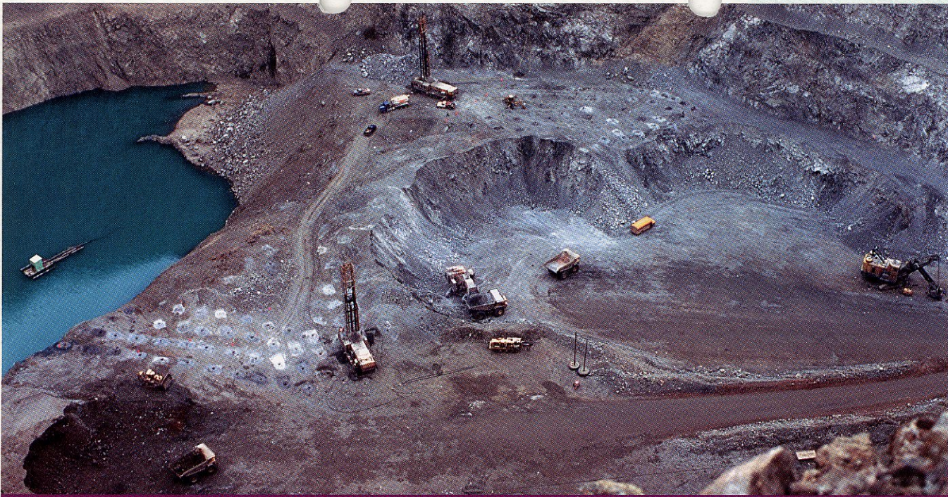
A successful drilling program identified reserves to allow development of the Ingerbelle Pit expansion.
