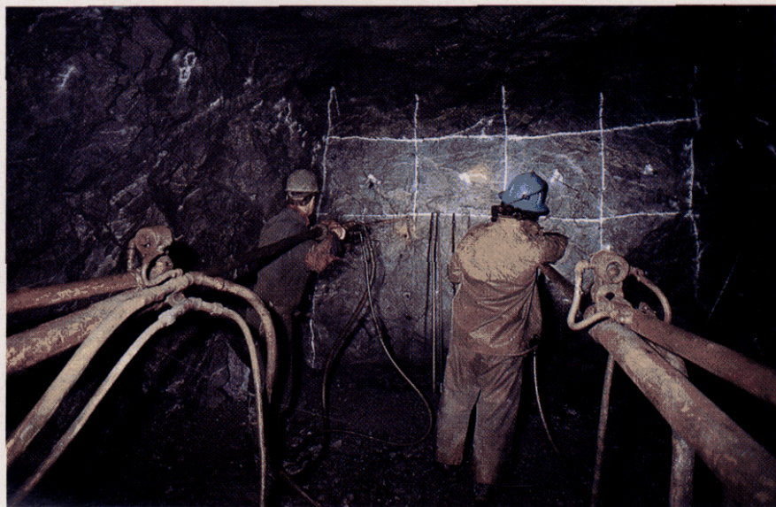
Drilling in a development heading underground.
