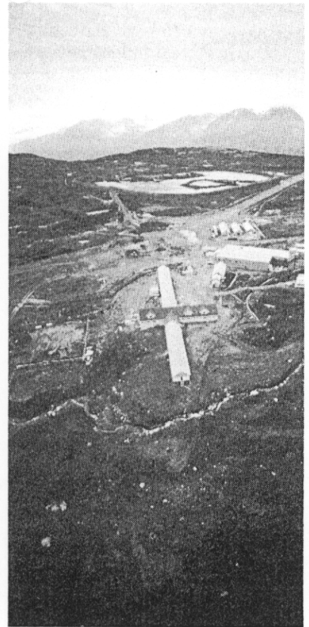
The Johnny Mountain mine, north-western B.C.
