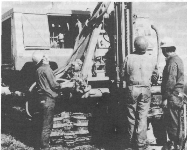
FIGURE 3. The Joy Manufacturing percussion drill mounted on a Nodwell muskeg tractor, used for scout drilling on the Red-Chris property in 1974 and 1975.
