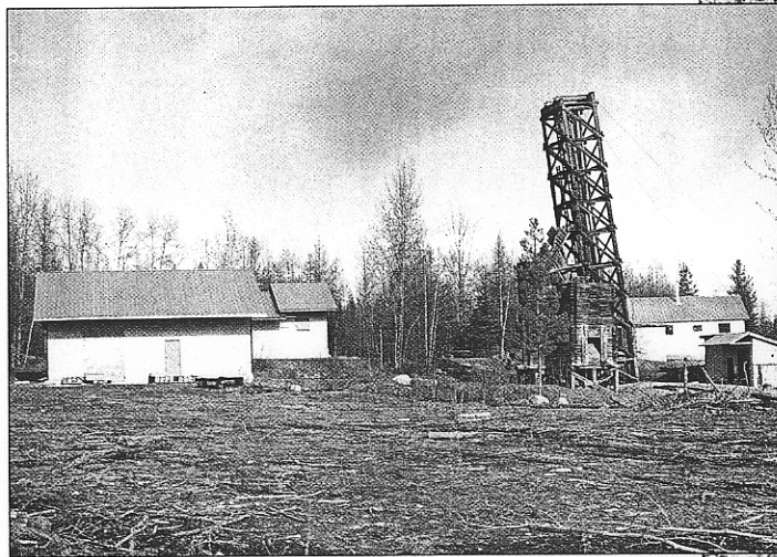
Surface facilities, Caramelia Project (Camp McKinney), Boundary Gold Fields.
