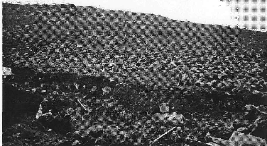
Ditching and trenching by hand is slow work. Courtesy: Randy Lord
