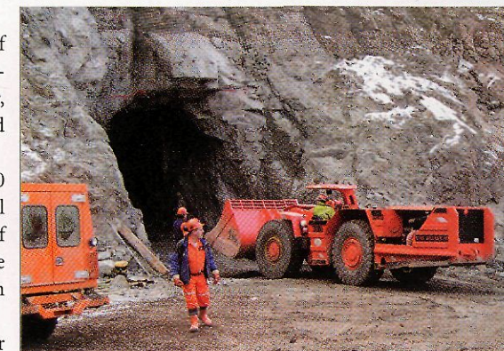
Richard Keane, shift supervisor from Procon Mining & Tunneling (left foreground) oversees continued work on an underground decline at the Afton copper-gold project in southeastern British Columbia. A 2-km decline is planned for the property, allowing drillers to complete 20,000 m of core from the underground workings, an effort designed to upgrade the measured and indicated resource to reserves.
