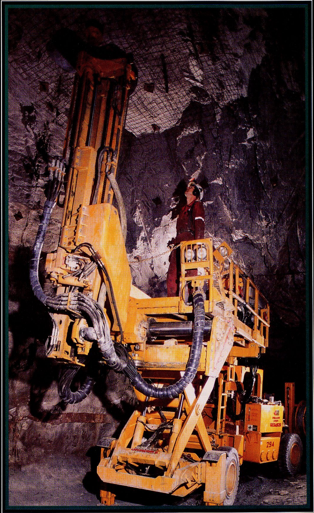
Rock bolter, H-W Mine, Myra Falls Operations
