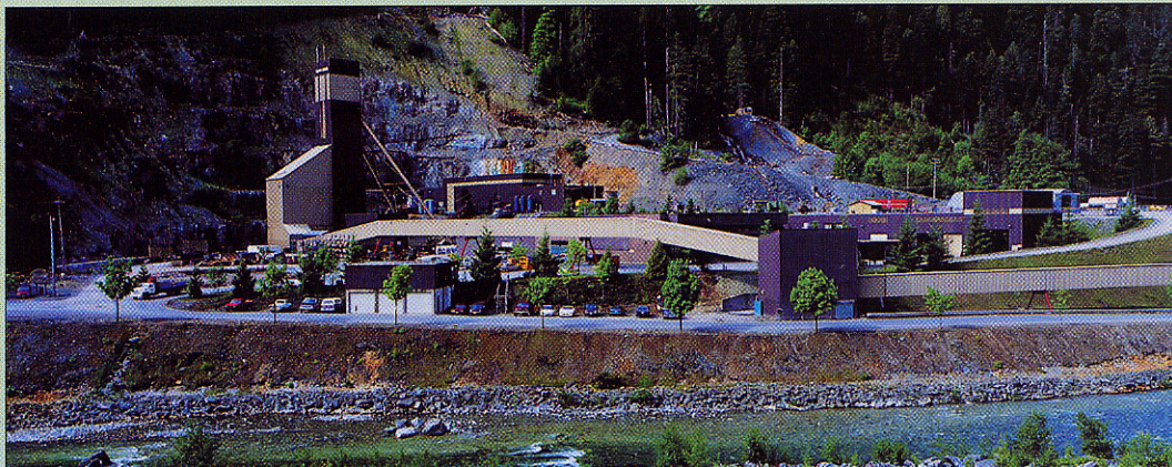
Surface facilities at the Myra Falls mine on Vancouver Island, B.C. The property produces zinc, copper and gold concentrates.
