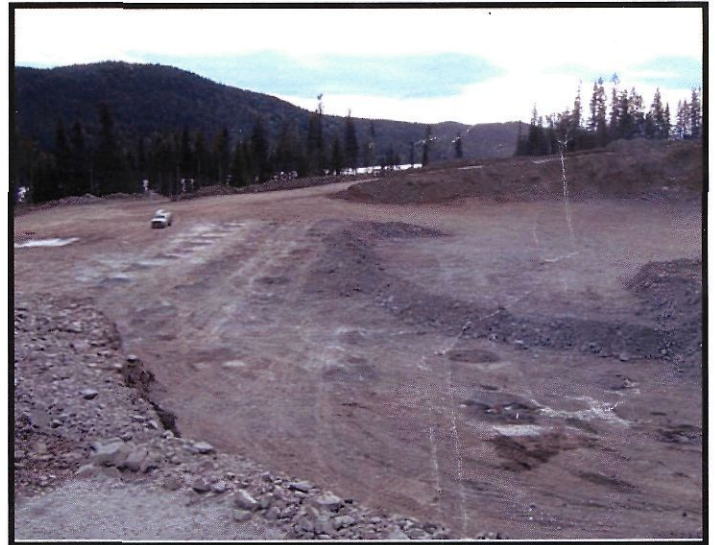
Drill holes WB1-WB2 looking south (Sept 2005)
