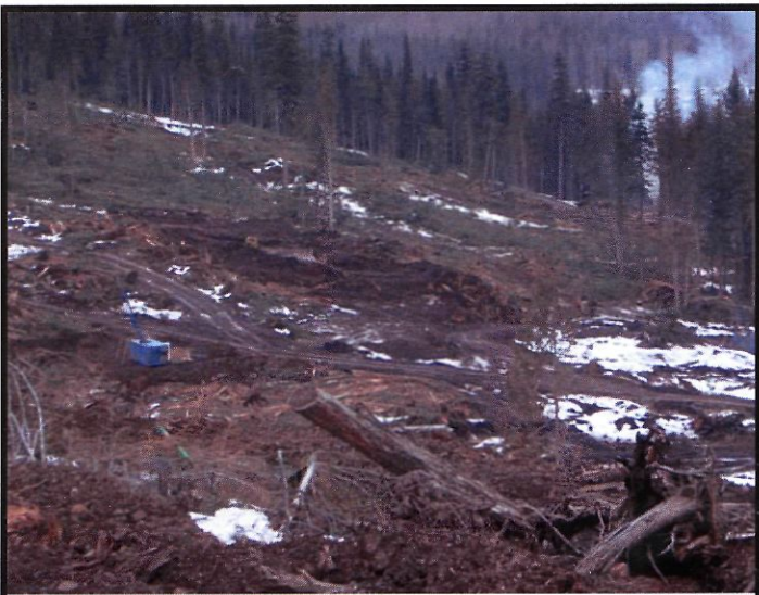
Preproduction drilling (Feb 05)
