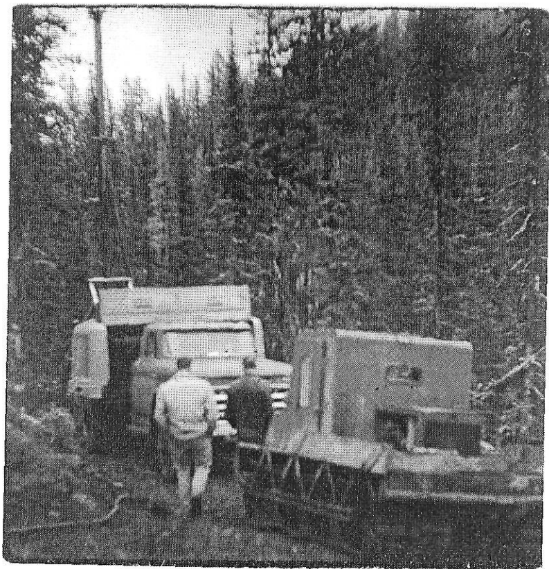
A TRUCK MOUNTED PERCUSSION DRILL WAS USED IN CONJUNCTION WITH SOME DIAMOND DRILLING IN 1946. THE RED BOMBARDIER WAS USED TO TRANSPORT MEN + SUPPLIES.
