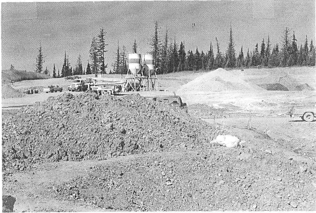
LOOKING FROM MILL AREA TO CONCRETE AGGREGATE SILOS
