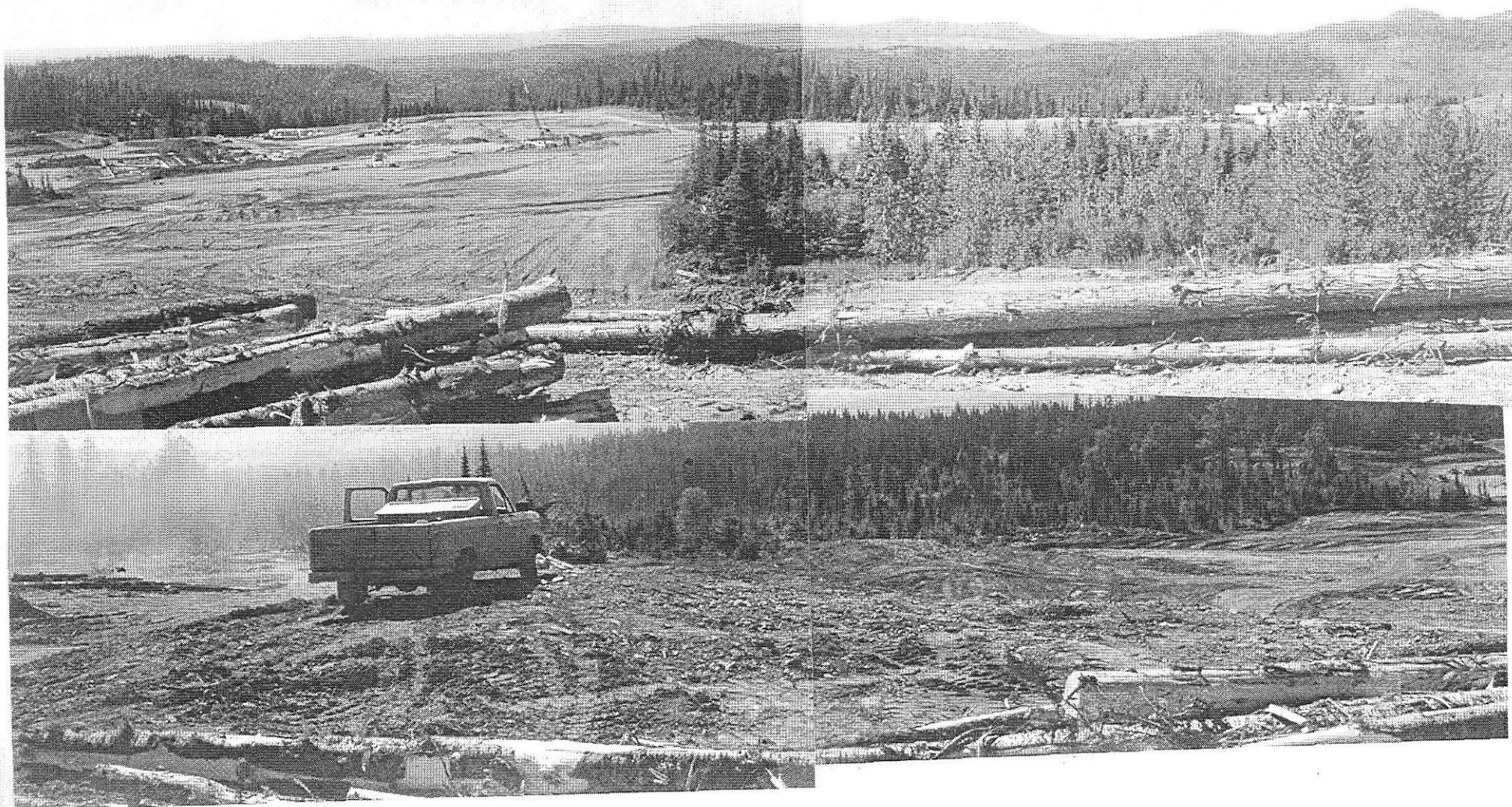
PANORAMIC VIEW LOOKING SOUTHEAST AND SOUTH OVER MILL FOUNDATIONS, CEMENT PLANT AND EQUIPMENT SHOPS.
